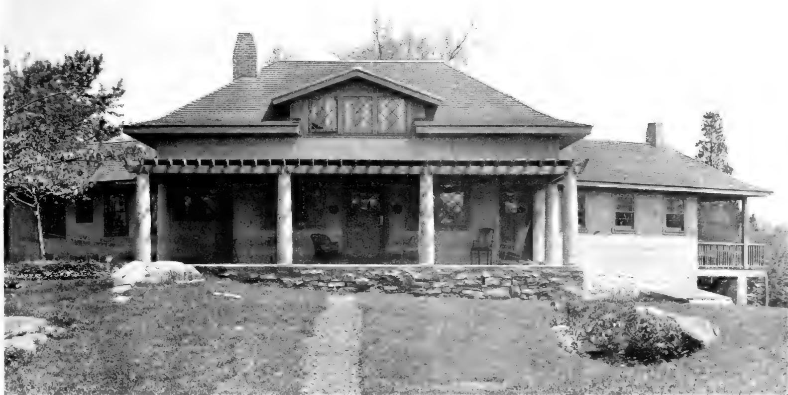
21—The House of Mr. Bassett Jones at Bryn Mawr Park, New York, has Reinforced Concrete Walls Finished with a Pebble Dash, and a Shingled Roof Stained a Moss Green with Good Effect
